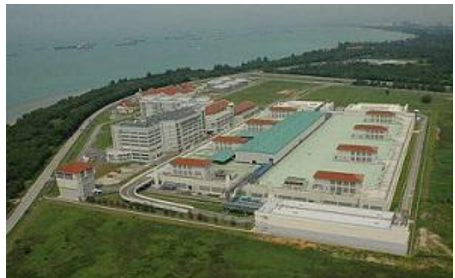
PUB@Changi Water Reclamation Plant
